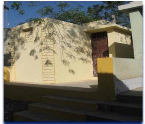
Well constructed Kitchen shed and in use at Sekhadiya Pra. Shala.
